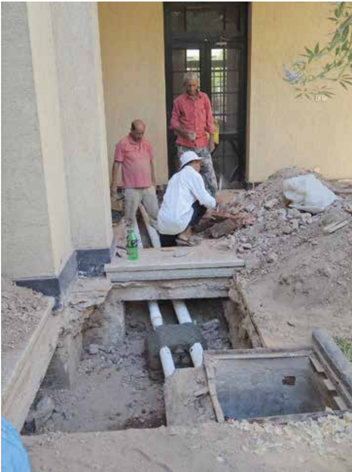
Courtyard plumbing project. Chicago House. September 2014. Photo by Tina Di Cerbo
