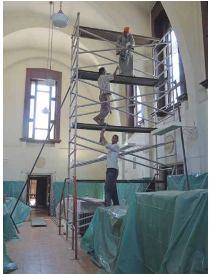
Repairing library shutters. Chicago House. September 2014. Photo by Tina Di Cerbo
