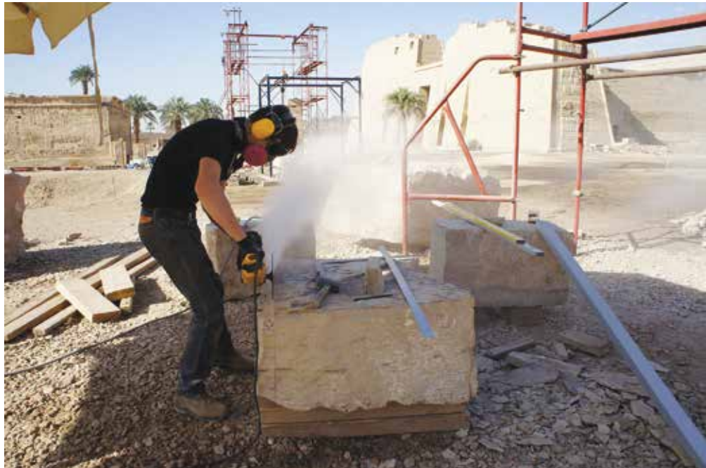
Johannes shaping stone for the Domitian Gate restoration. Medinet Habu. Photo by Ray Johnson
