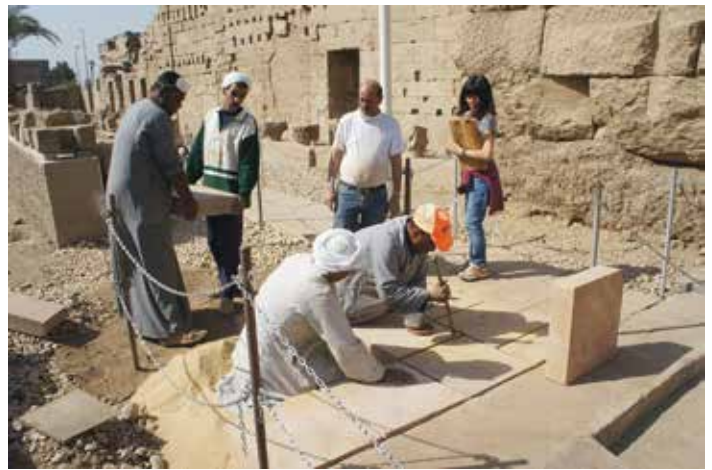
Building the access ramp. Luxor Temple. Photo by Ray Johnson
