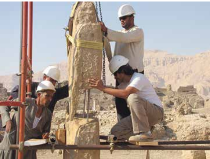
Well roof-block joining. Medinet Habu. December 2014. Photo by Nahed Samir
