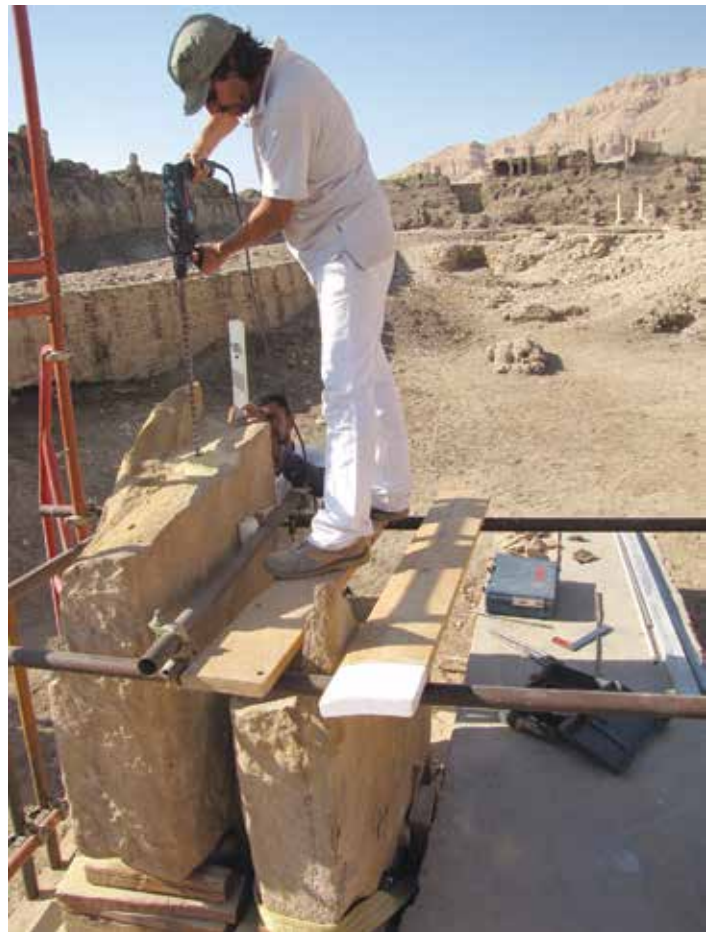
Well roof-block joining. Medinet Habu well . December 2014. Photo by Nahed Samir
