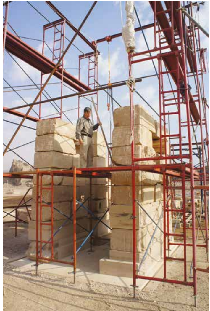
Frank checking block placement. Medinet Habu Domitian Gate. December 2014. Photo by Ray Johnson
