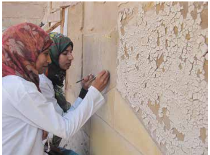
Conservation students desalinating exterior western wall, small Amun Temple. Medinet Habu. Photo by Lotfi Hassan
