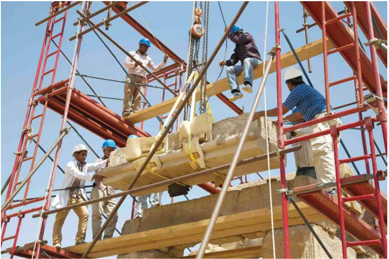
Raising Domitian Gate cornice during Minister's visit. March 22, 2015. Photo by Yarko Kobylecky
